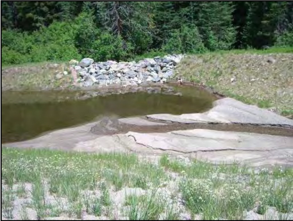
Typical Collection site – Basin
